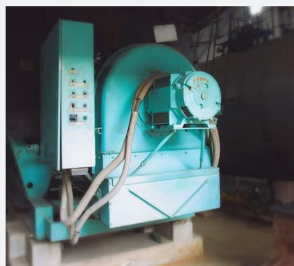
Economizer Boiler raises the boiler feed water temperature, lowering the needed energy input, reducing the rated boiler output's firing rates. Our boiler feed tank is adequately insulated to maintain the feedwater temperature above 90°C at all times. Moreover, we are using a built-in economiser in the boiler that recovers heat from exhaust gases, which transfers this to the incoming boiler feed water, thus increasing the overall boiler thermal efficiency and reducing CO2 emissions.
